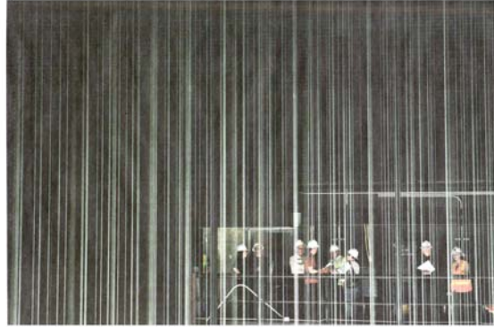
Light glances off dozens of rows of cables strung above the performance space at the Wyly Theatre, used to "fly" scenery up and out of sight.
